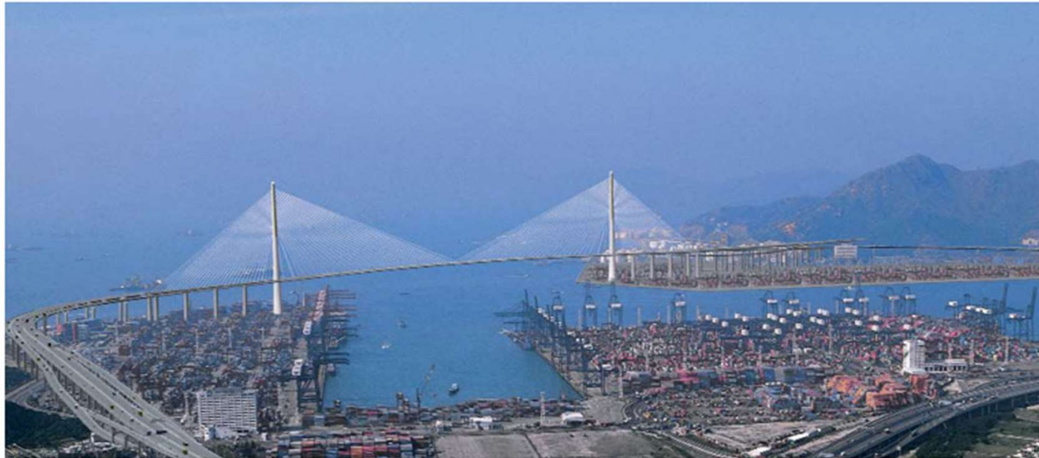
Stonecutters Bridge, Hong Kong, Čína, 2010
